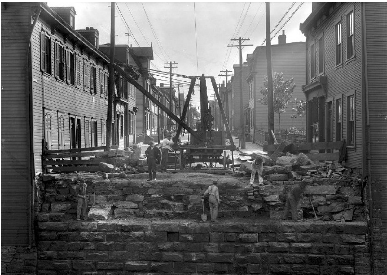
Lowrie Street Bridge. August 31, 1915. Pittsburgh City Photographer Collection, 1901-2002. Description of view: Workers cutting down the old abutment on the Lowrie Street Bridge.
