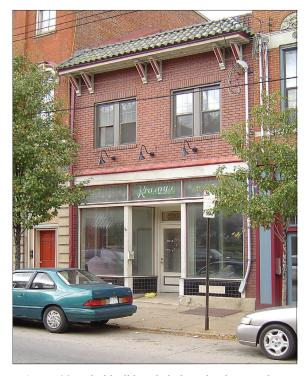
Figure 22. Tiled bulkheads below display windows
