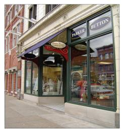
**Figure 10.** Storefront set in structural frame
