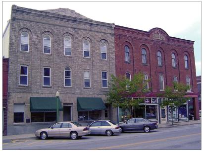
**Figure 23.** Commercial building with inappropriate synthetic stone on brick facade
