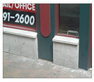
Figure 21. Stone bulkheads below display windows
