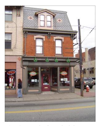
Figure 27. Mansard roof restored with slate
