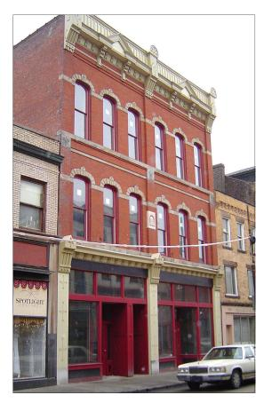
Figure 24. Brick façade cleaned and repointed
