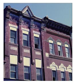
Figure 28. Inappropriately small replacement windows
