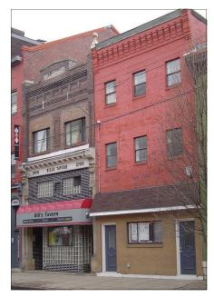
Figure 6. Inappropriate remodeling: closing up storefronts and windows, covering transom windows
