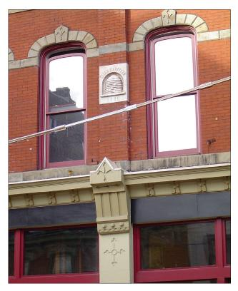
Figure 25. Stone trim cleaned and repaired
